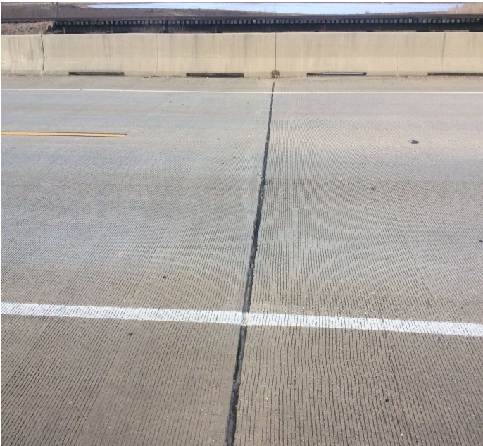
PHOTO 1 Description Joint - Bent 2 (material losing adhesion)
